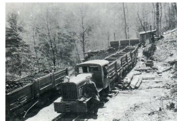
The narrow gauge gasoline locomotive with a string of one-ton ore cars. [David Sams]
