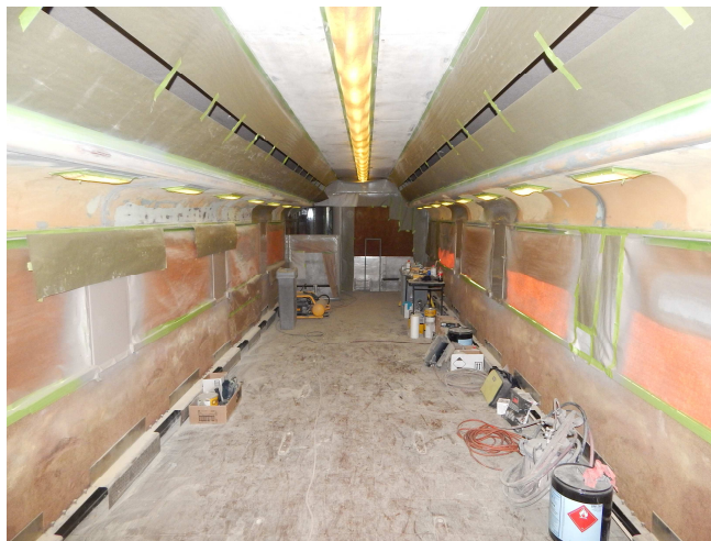
View of interior painting work on the 539 at NCTM.
