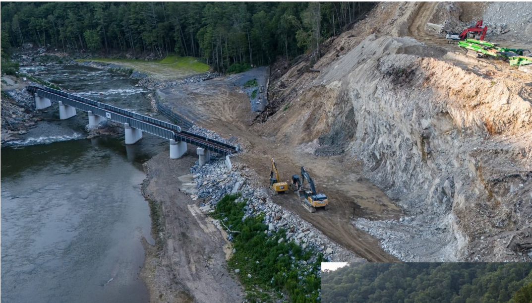
Poplar RoW Realignment. 8/14/25 The quarry here has been ordered to stop working, but crews are still chipping away at the mountainside to reduce the curvature coming off the bridge at Poplar.
